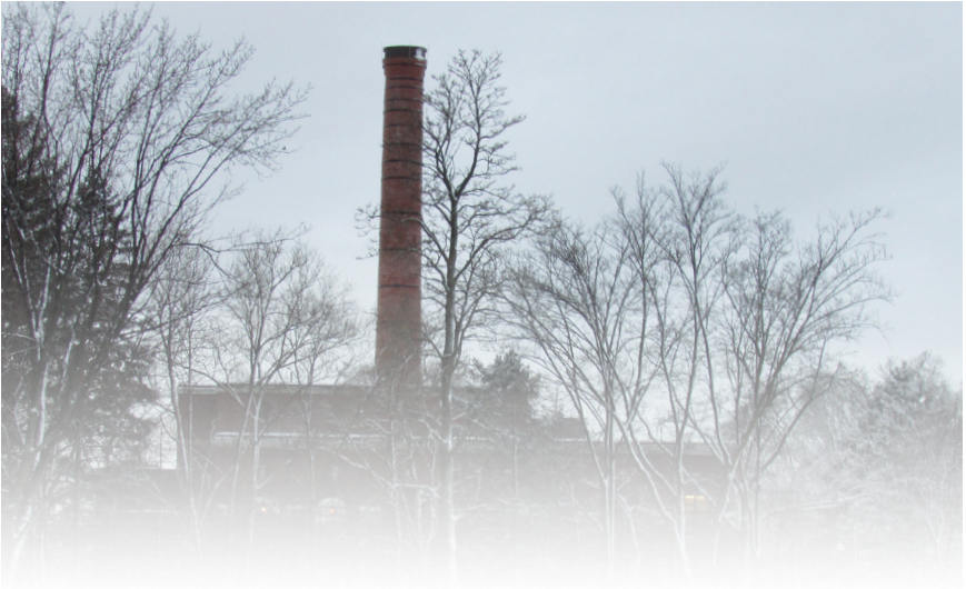
The Powerhouse Jim Tate, 2019
